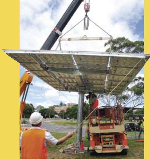
Left: the CPV array tracks the sun during the day, and above, is lowered into place during construction
